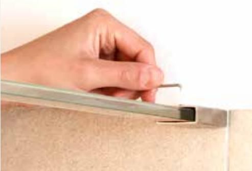
Insert the set screw and tighten at the tiled wall end.
