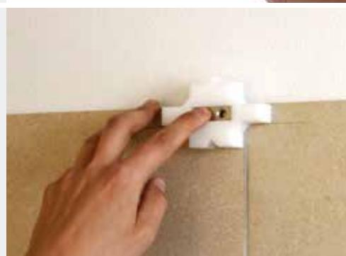
Press the wall bracket against the tiles through the hole in the foam block. The foam block will hold the bracket in place while the glue dries.
